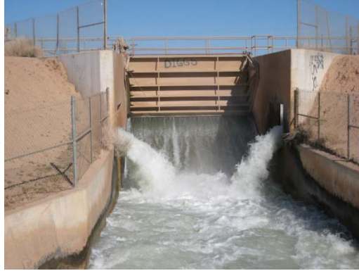
Maricopa-Stanfield Irrigation District Drop Structure; 100 cfs; 10 feet head; 200 kW potential
