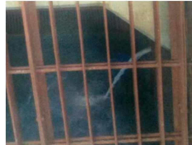
Leak Reduced 11-04-04 Leak Sealed 11-04-06 Sodium Silicate Injection
