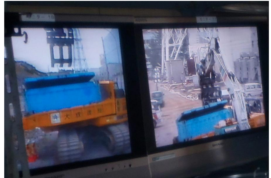
Remotely Operated Construction Equipment Reducing Gamma Field and Debris Removal
