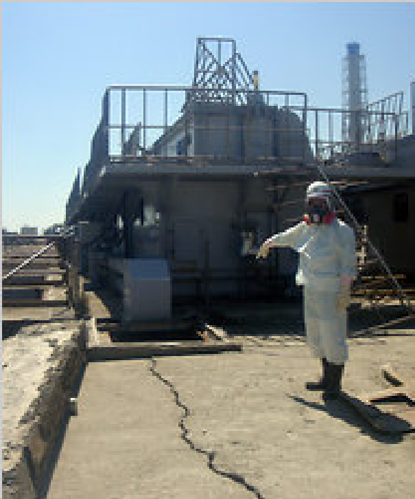
Non-Safety Grade intake Structure
