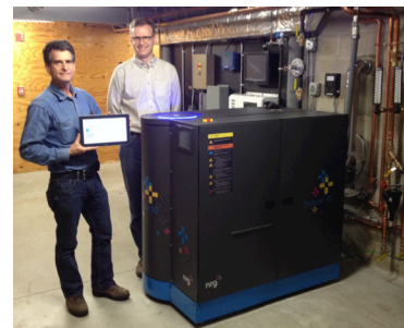
Figure 3: Example of an advanced CHP system developed by Dean Kamen of DEKA Research and Development. (Photo by G. Morgan.)
