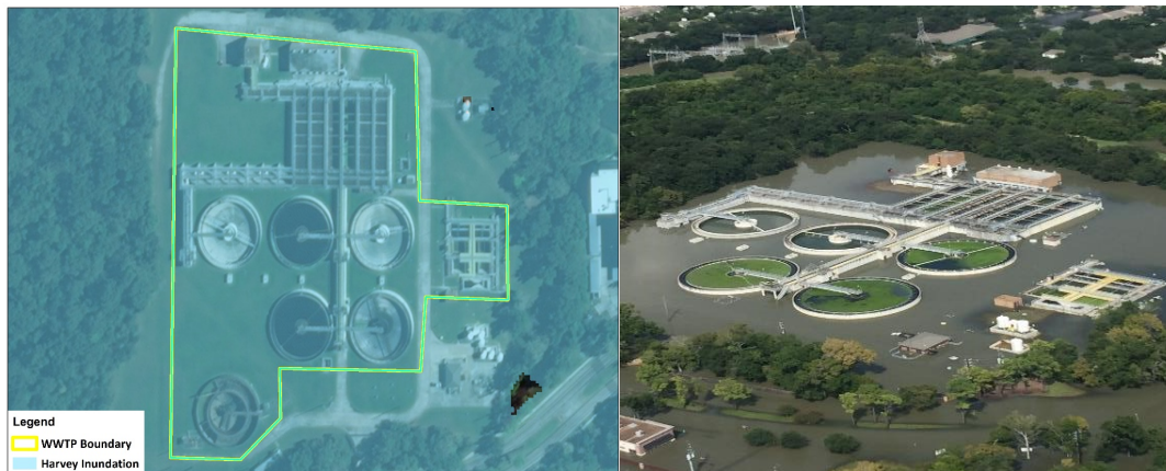
Figure 9. Illustrations of the modeled extent of flooding from geospatial modeling of wastewater treatment plants after Harvey (select facilities shown in the top figures). The bottom images compare the modeled flooding during Harvey on the left to an actual photograph taken during Harvey on the right for the Turkey Creek wastewater treatment plant
