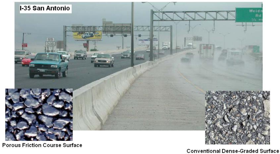
Figure 2. Porous Friction Course Surface (left) Compared to Conventional Surface (right) After a Rain Storm.
